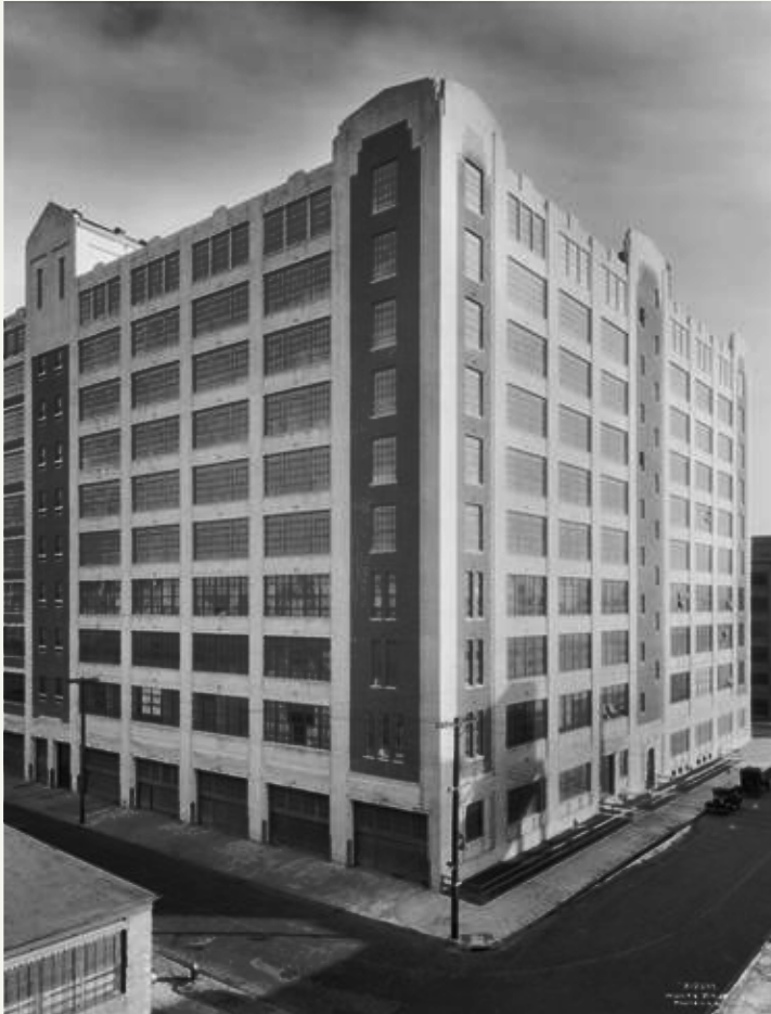
The Factory ca 1930 as the former R.H. Macy and Co. warehouse
